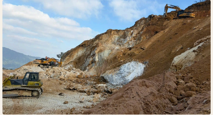
Selective blast — controlled lump size for batching
